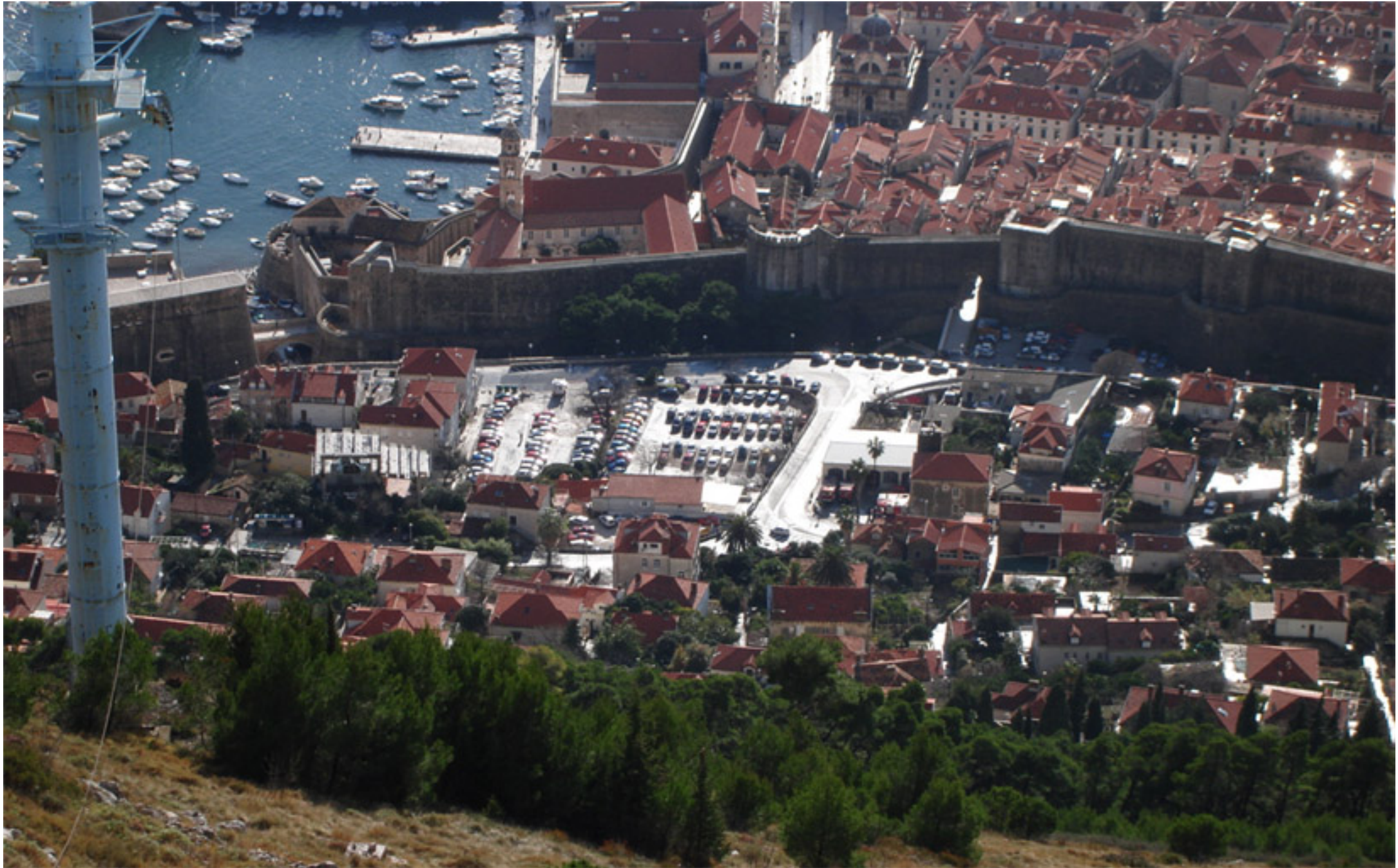
A - View of the site from the cableway
