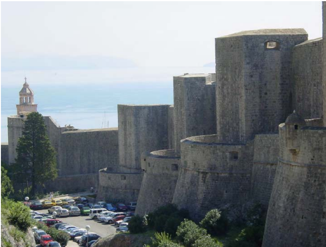
A - View of the city walls from the north
